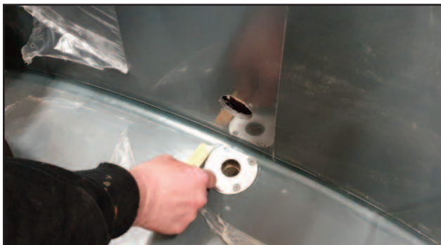
10. Wipe away any excess silicone. Insert the 4 screws:
